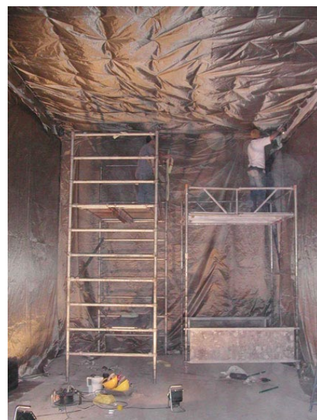
T-Mobile chamber in Bonn, Germany (under construction)
